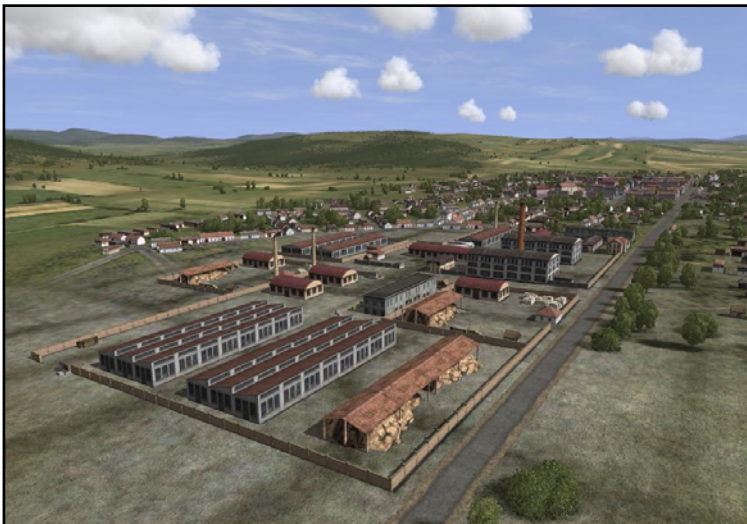
Zlin Footwear and Tyres Factory Baťa Zlín – továreň na obuv a pneumatiky Location: A-12 num 8 Altitude: 20 m
