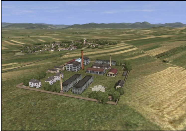
Lietavska Lucka Cement Works Cementáreň Lietavská Lúčka Location: I-12 num 1 Altitude: 70 m
