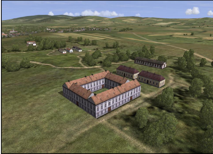
Hlohovec Chateau Hlohovský zámok 12th century (last rebuilding 18th century) Location: B-3 num 7
